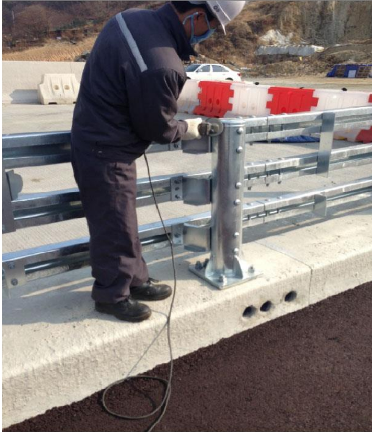
POST CAP-WELD-GRIND
